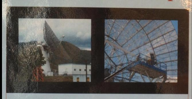
Construction began on this telescope in 1959 and was completed in time for the official opening of DRAO in 1960. The dish is 25.6m in diameter, fully steerable, has an open-mesh surface, and can observe at multiple frequencies.
